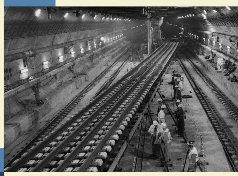
Line: London – Paris Length of LVT slab track: 100 km / approx. 310'000 supports Design axle load: 22.5 t Design speed: 200 km/h Traffic: Passenger and freight trains
