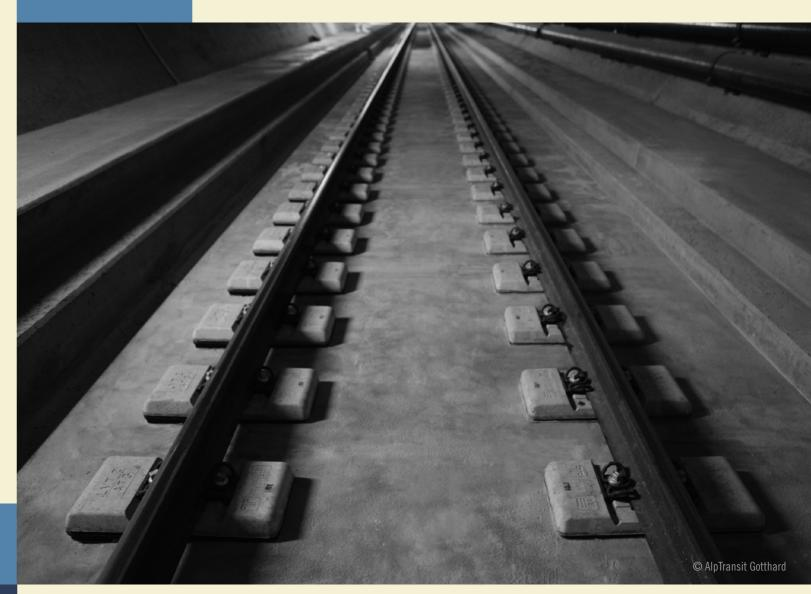
Line: Zurich – Milan Length of LVT slab track: 114 km / approx. 380'000 supports Design axle load: 25 t Design speed: 250 km/h Traffic: High-speed and freight trains
